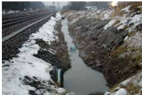
This is the result of a complete culvert refurbishment.
